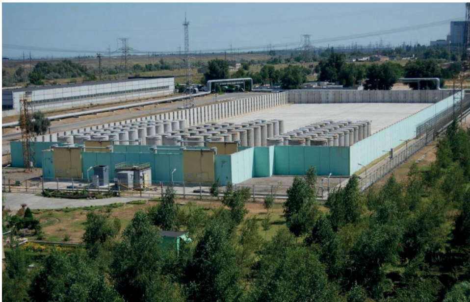
Dry spent nuclear fuel storage. Photo: Energoatom
