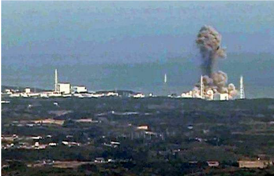
Explosion of a hydrogen mixture at one of the reactors at the Fukushima nuclear power plant. Photo: TV screenshot
